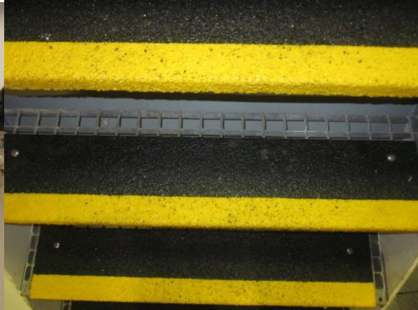
Anti-slip plates fitted to another set of stairs.
