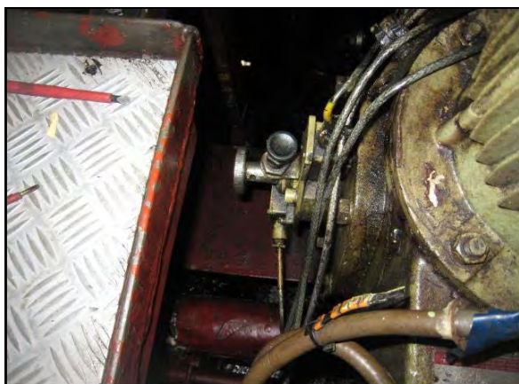
Machinery Space for cam shaft inspection
