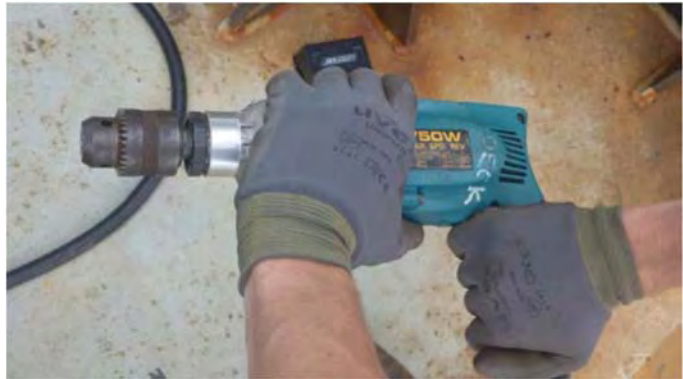
Hand Positioning whilst drilling hole
