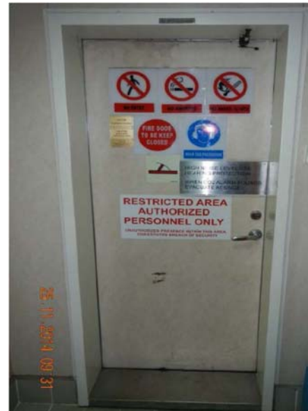
Engine room access door
