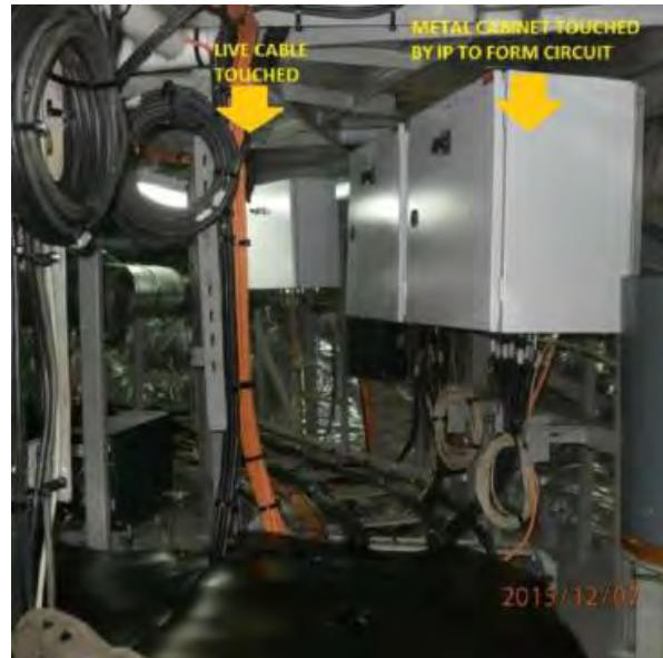
IP place hand on live cable and metal cabinet, forming a circuit
